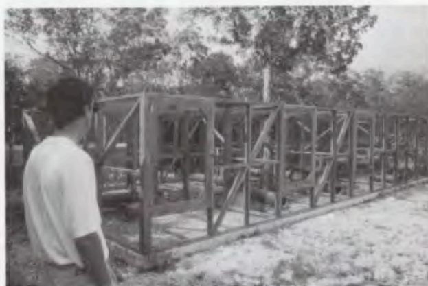
The first captive facility built in the Botanic Park shown at completion in 1996. The facility was funded by Milwaukee Country Zoo and its partner Foundation for Wildlife Conservation. The facility included 12 8 x 8 foot and 16 4 x 4 foot cages. Photographer unknown.
